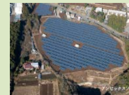
Operation of Mega Solar Powerplants
