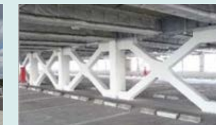
Seismic reinforcement (Kokudo BuilACE Company)
