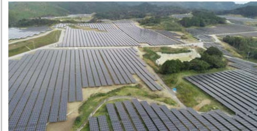
Capacity : 42.0MW Earthwork Scale : 544,100m 3 Completion : July 2019
