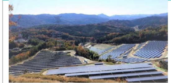
Capacity : 25.4MW Earthwork Scale : 1,100,000m 3 Completion : October 2019
