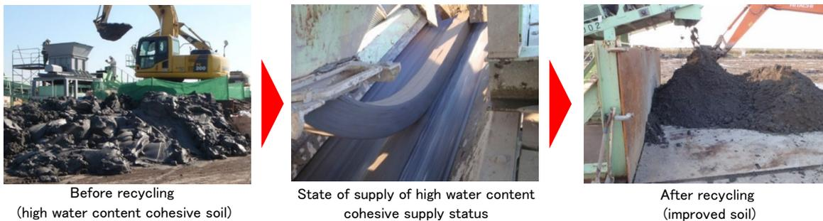
■ Recycling of soil containing underground stems: Removing underground stems from high water content cohesive soil mixed with underground stems for effective use
