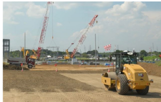
Actual use of automated construction systems
