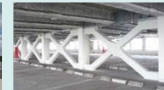
Seismic reinforcement (Kokudo BuilACE Company)
